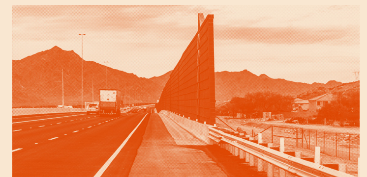
FIG. 11 - Loop 202 South Mountain Fwy via AZDOT
